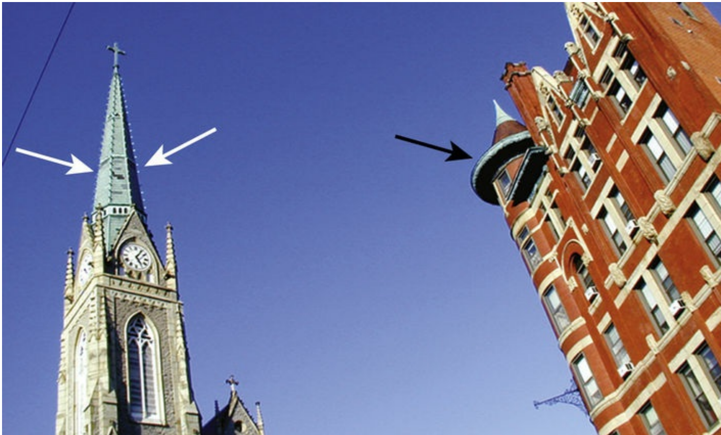
• FIGURE 2-3 Steeple sign.
